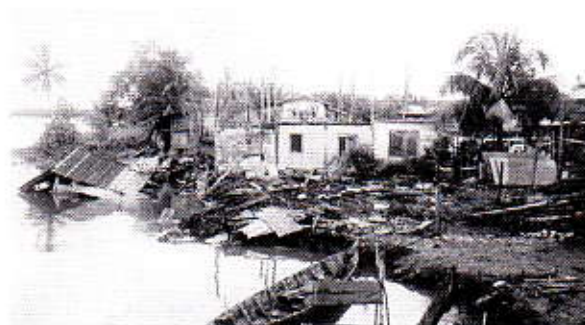
The remains of the 6 houses that were swept away by the strong current.
