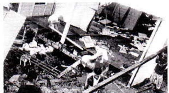
Trying to salvage whatever building materials they can get hold of so that they can reuse it to rebuild their houses.
