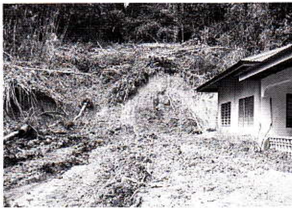
Part of the section where the landslide caused damages.
